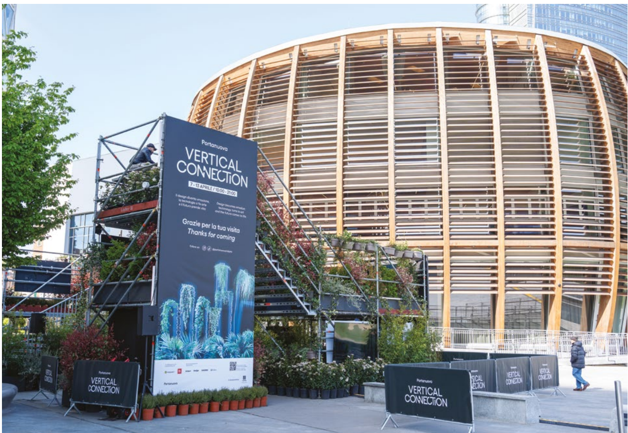
Portanuova Vertical Connection, in piazza Gae Aulenti
